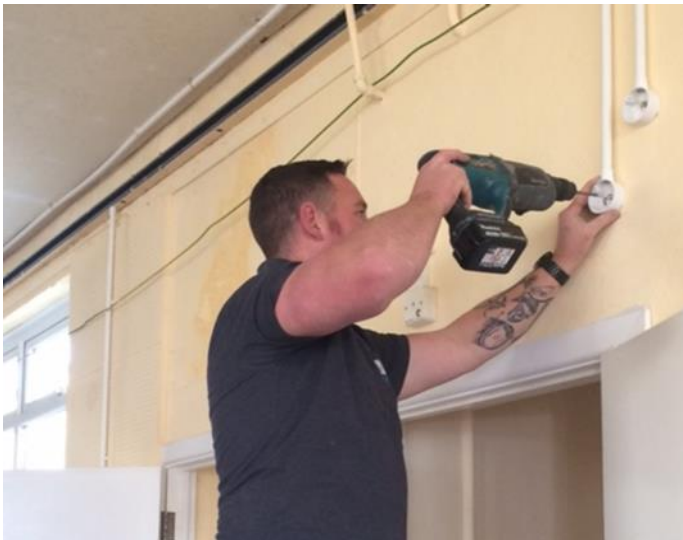
Simon tackling the mammoth task of rewiring the building
