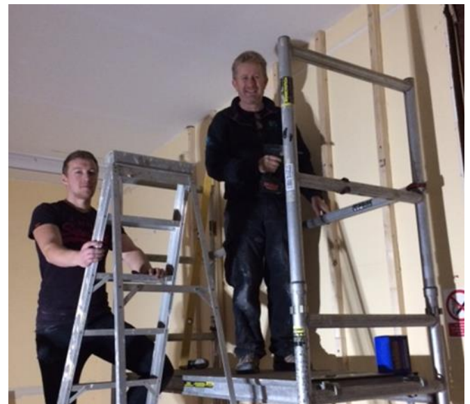
Steve and Jude cracking on with building work
